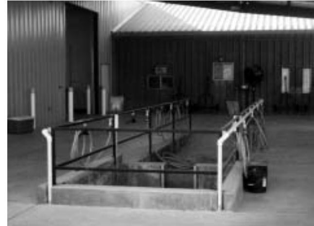
The redesigned and greatly improved wash pad at Prairie Dunes Country Club provides adequate collection and filtering of wash water.
