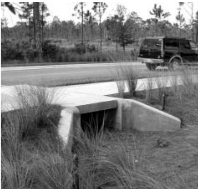
A tunnel under a road at Pelican Preserve provides safe passage for wildlife.
